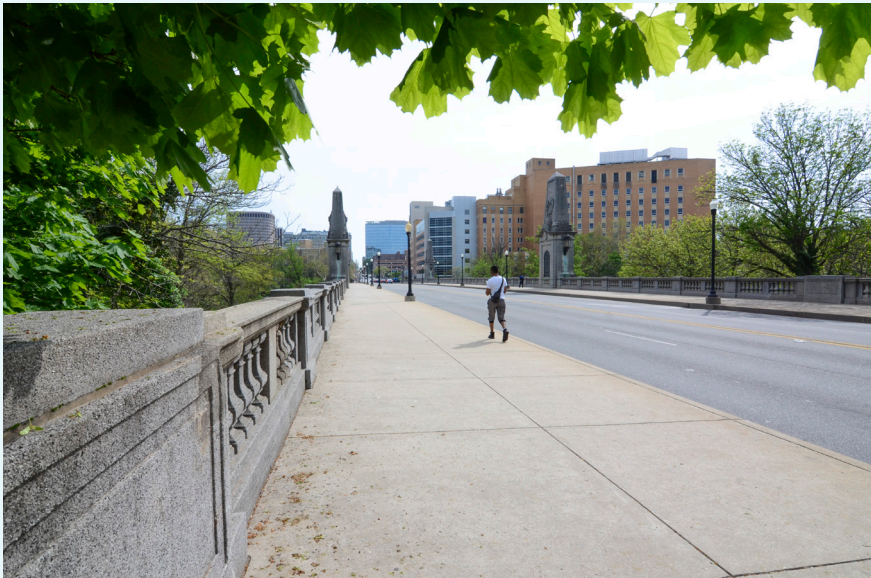
The Washington Street Bridge, which connects the community to Downtown Wilmington.
