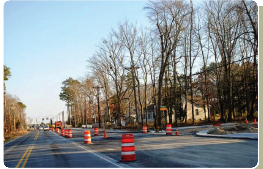
SR 54 Road Improvements Credit: Lee Cannon
